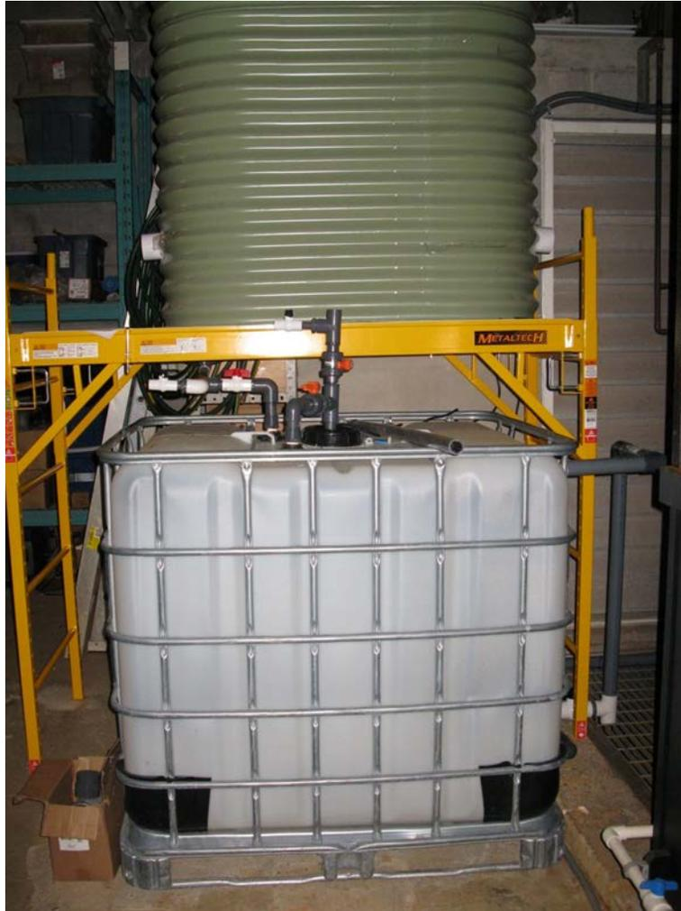
*Figure 3.* Bioreactor technology configuration for Fleming College salmon hatchery experiment. The green metal housing contains the membrane placed atop the 1000L tote containing the wastewater. (Photo credit: Centre for Alternative Wastewater Treatment, 2013).
