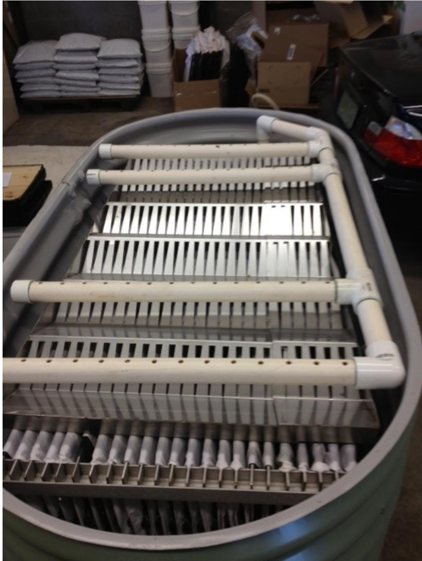
*Figure 2.* The wastewater dispersal piping located on top of the membrane in the bioreactor housing unit. (Photo credit: Centre for Alternative Wastewater Treatment, 2013).
