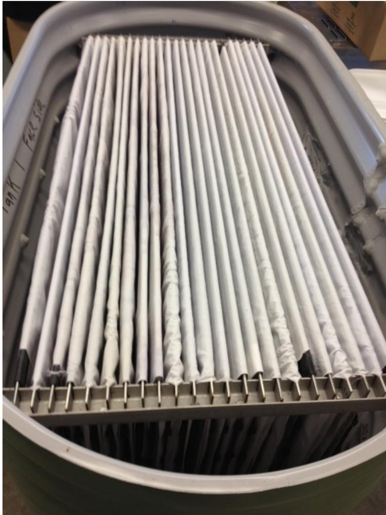
*Figure 1.* Photo of the Biogill® bioreactor membrane suspended in the housing unit. (Photo credit: Centre for Alternative Wastewater Treatment, 2013).
